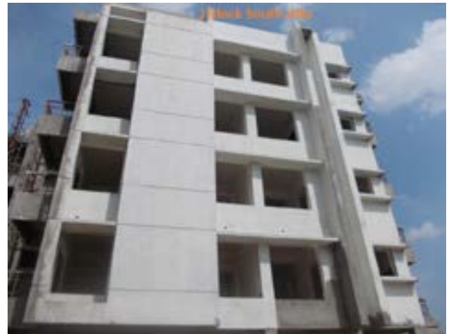
South Side of Block J
